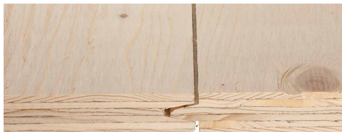
Figure 16. Tongue and groove (TG) joint
