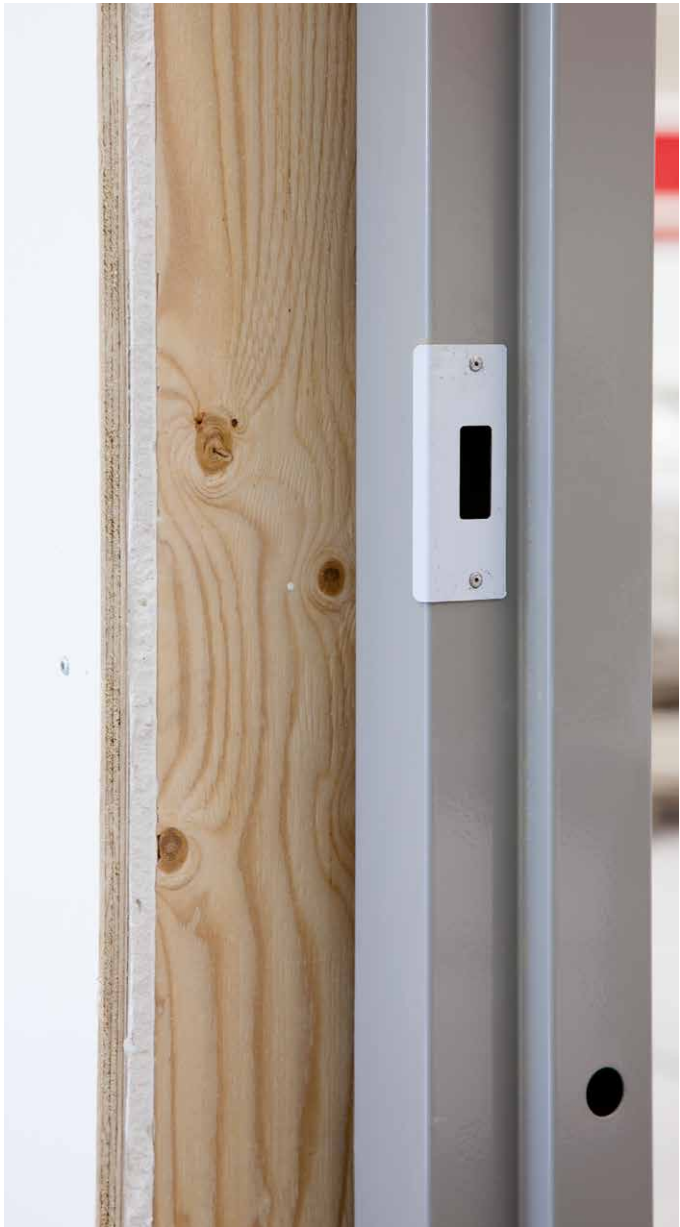
Figure 33. Spruce Flex is used to protect gypsum board wall
