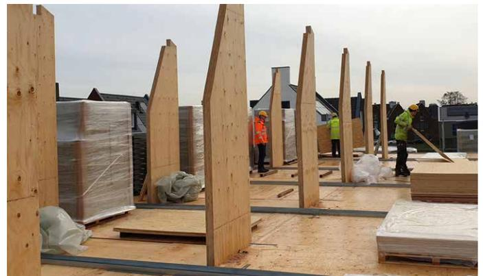
Figure 1. Machined Kerto LVL components
