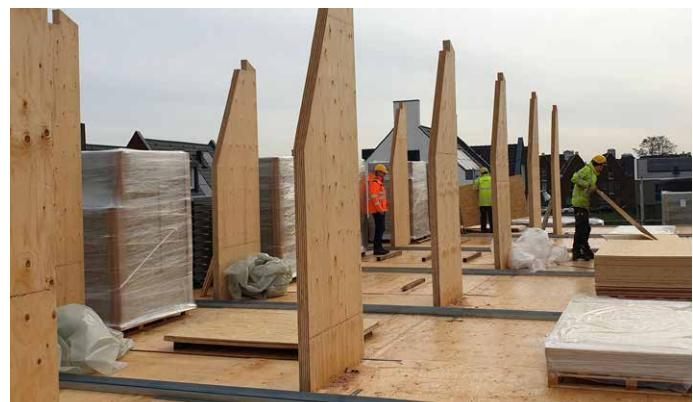
Figure 1. Machined Kerto LVL components
