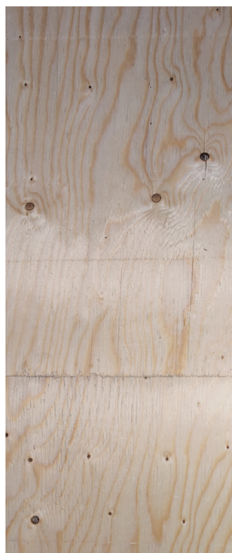
Figure 2. Front side, unsanded, light colour glue in scarf-joints
