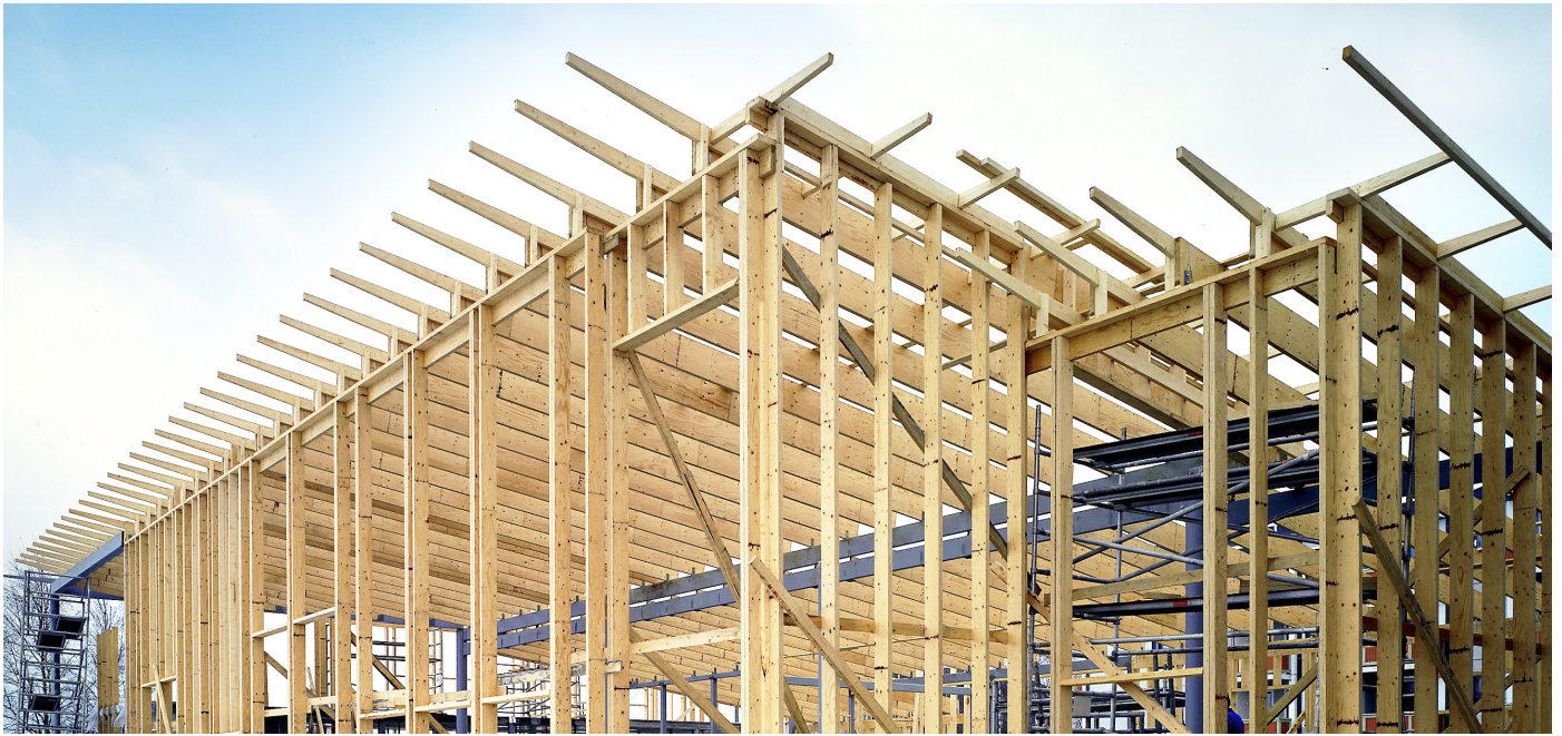
Figure 4. Kerto LVL as framework studs
