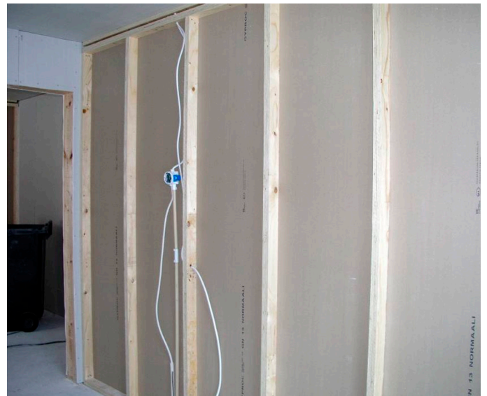
Figure 5. Kerto LVL studs in partition walls
