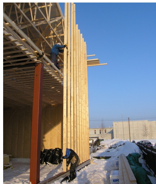
Figure 3. Kerto LVL studs in exterior walls
