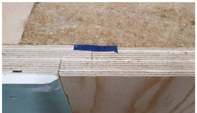
Q-panel with half-lap with insulation and adhesive tape.
