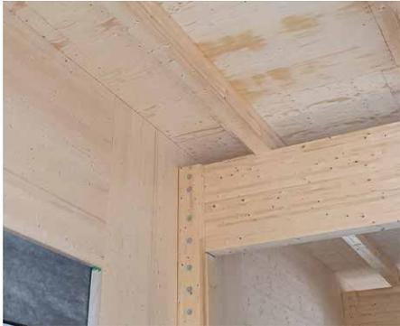
Kerto LVL Q-panel with half-lap used in roof panelling.
