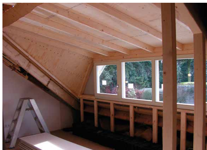
Figure 55. Dormer structure from inside
