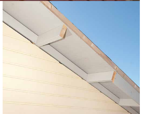
Figure 24. Cantilevers supporting eaves overhang
