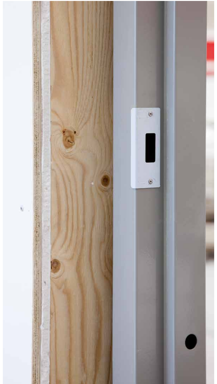
Figure 33. Spruce Flex is used to protect gypsum board wall
