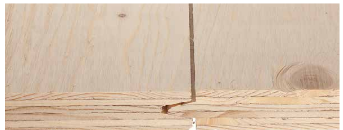
Figure 16. Tongue and groove (TG) joint
