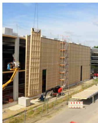
Brüninghoff, Germany 13 m high wall elements
