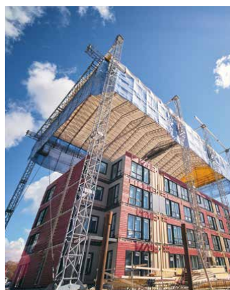
Linnanfältti, Finland Efficient off-site construction with wooden elements
