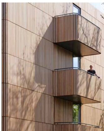
Monicahof, Netherlands Sustainable, safe and material-efficient residential building
