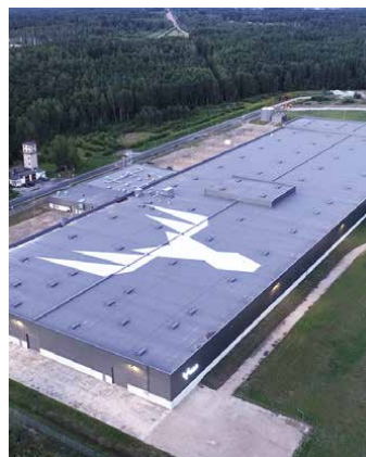
Metsä Wood Pärnu mill, Estonia Fast construction with wooden roof elements
